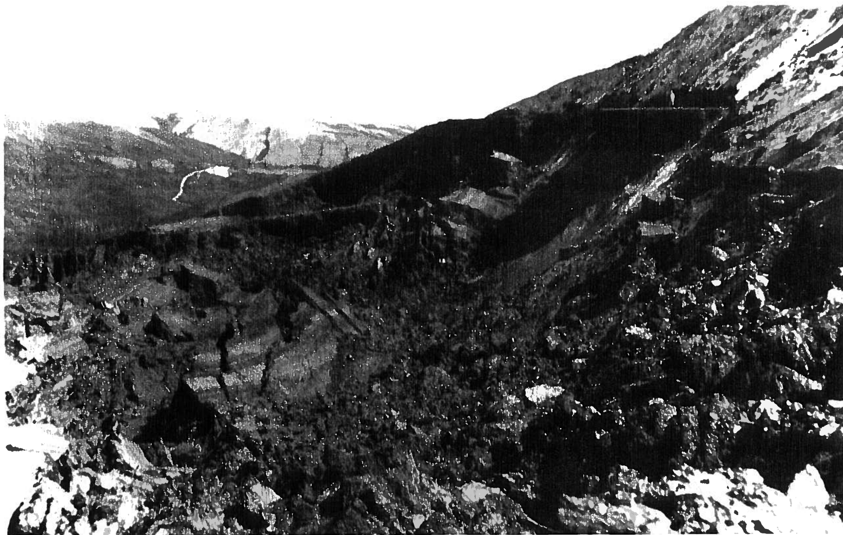
Fig. 4 Looking south into slide escarpment. Man standing on original highway grade.
