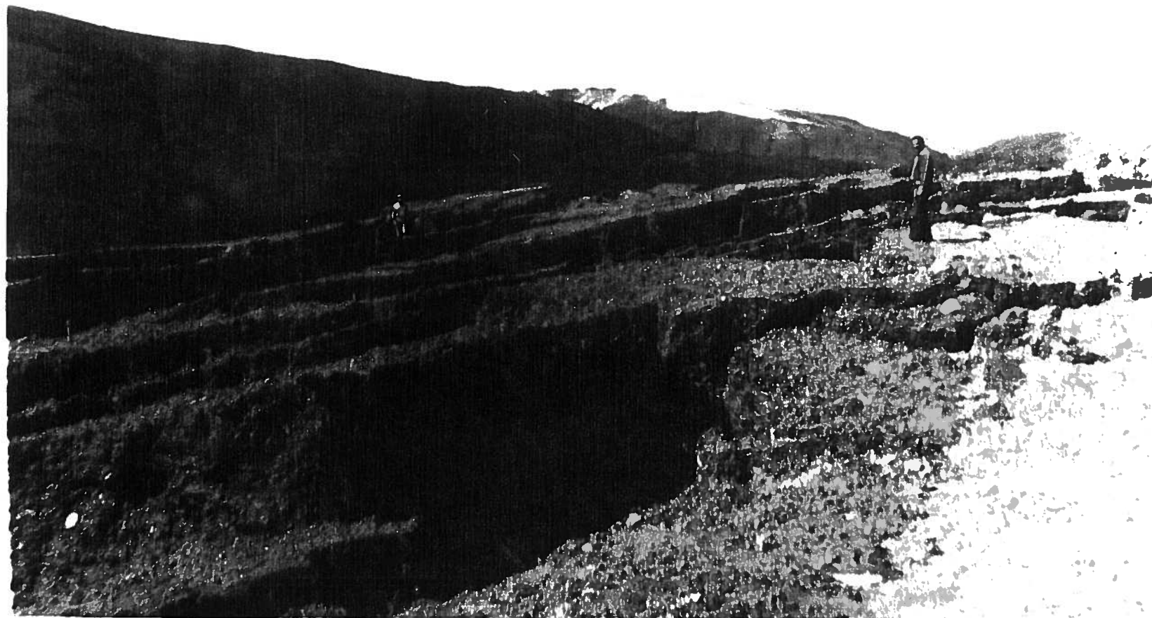
Fig. 5 Looking south over slide. Material shown was fill for highway grade.
