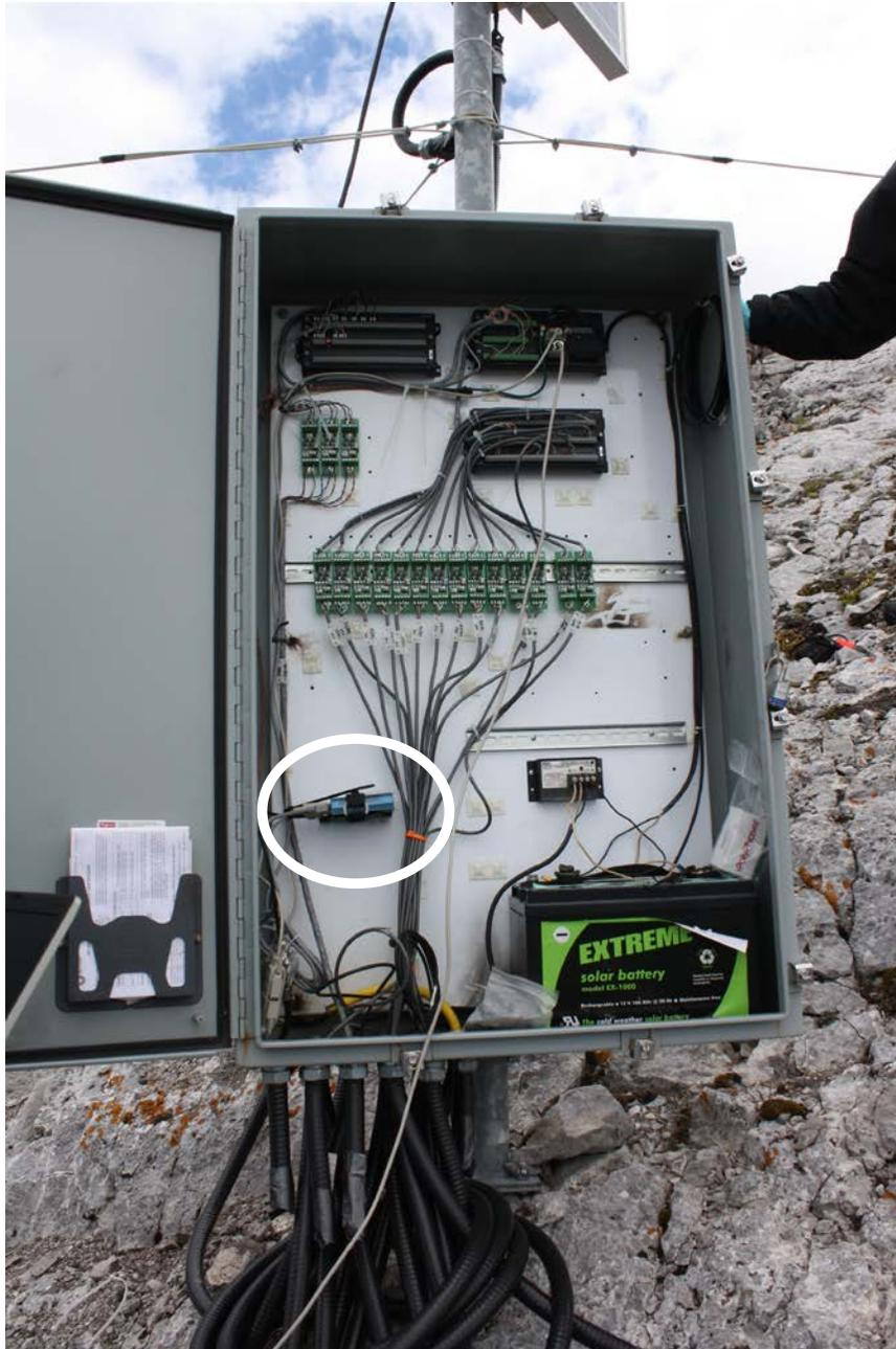
**Figure 3. Physical layout of equipment installed at the borehole datalogging site on Turtle Mountain, southwestern Alberta. Cellular modem can be seen in the lower left (white circle).**
