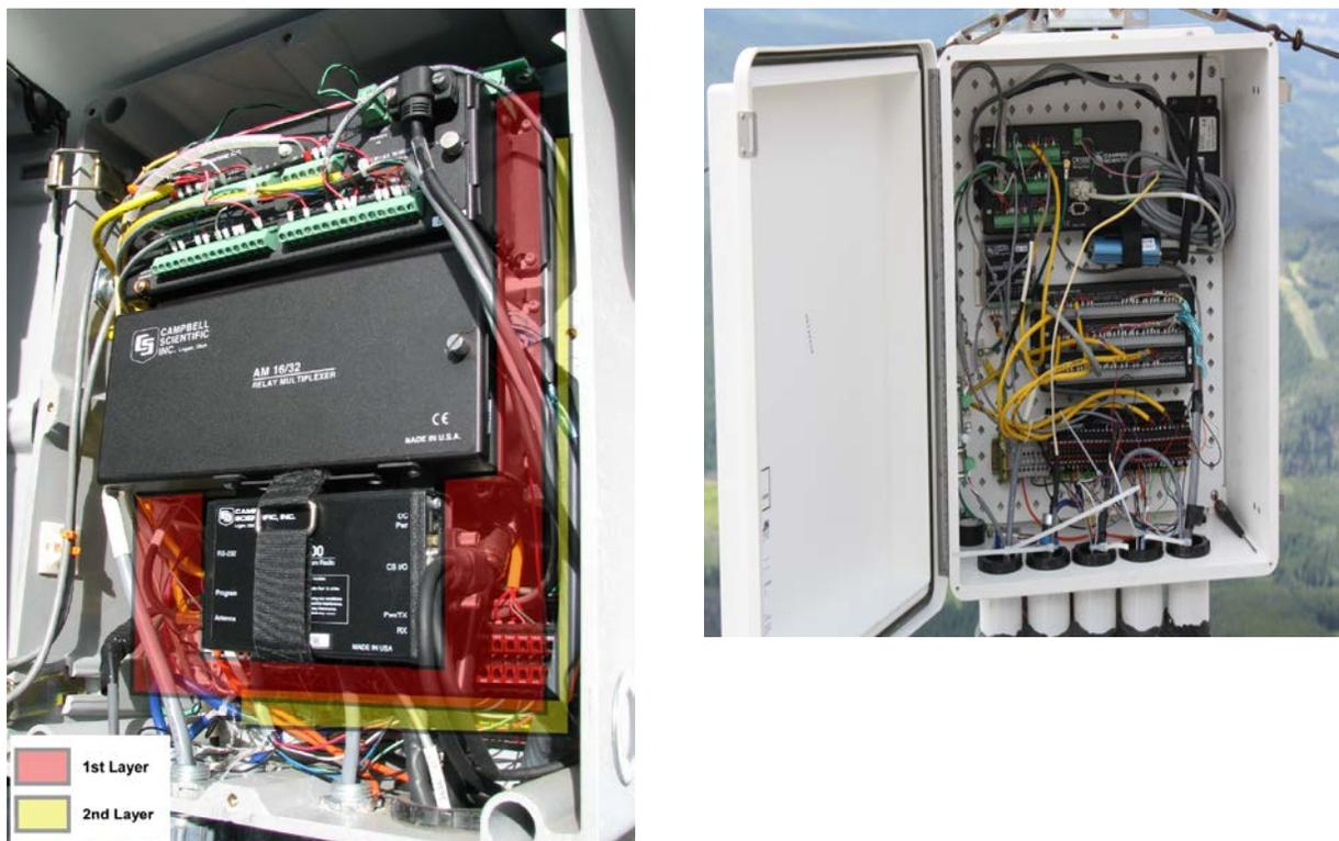
**Figure 4.** Physical layout of equipment installed at weather station datalogging site on Turtle Mountain, southwestern Alberta. Limited space in the old enclosure (left) made repair work difficult. The new enclosure (right) is a significant improvement because all equipment is now in a single layer.
